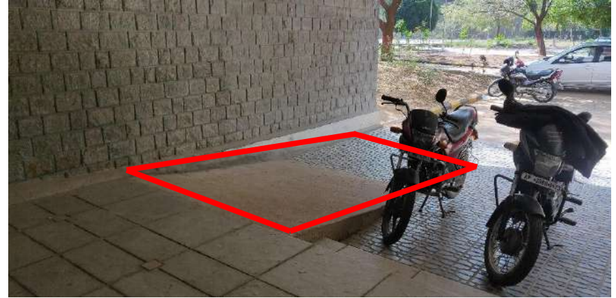
RAMPS LEADING TO PLINTH LEVEL FROM PARKING SIDE WITH A SLOPE OF MIN. 1:12
