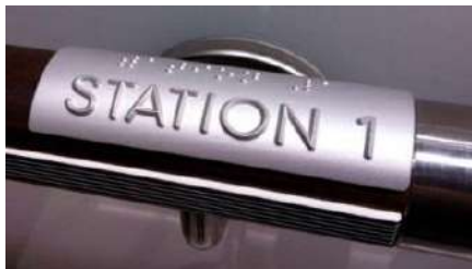
Braille signs on handrails
